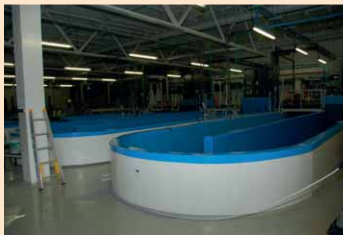
Foster-Lucas tanks combine the advantages of a circular tank (better circulation of water) with those of a raceway (better surface area to floor space ratio).
